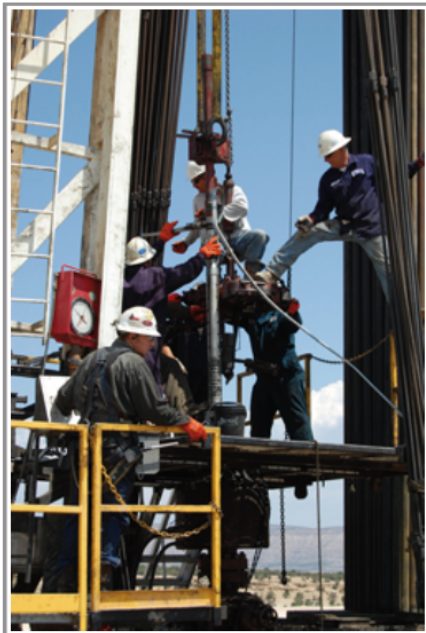
Fig 1. AWS downhole installation.
